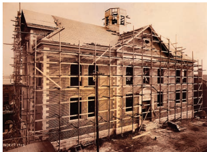
The Jonathan Bourne Whaling Museum is seen under construction in this silver gelatin print dated Nov. 27, 1915 from the Benjamin Baker Collection. The west-facing palladium windows in the rear of the Old Dartmouth Historical Society's Rogers Building are visible in the lower left corner of the photograph. NBWM 2000.100.89.3.326
