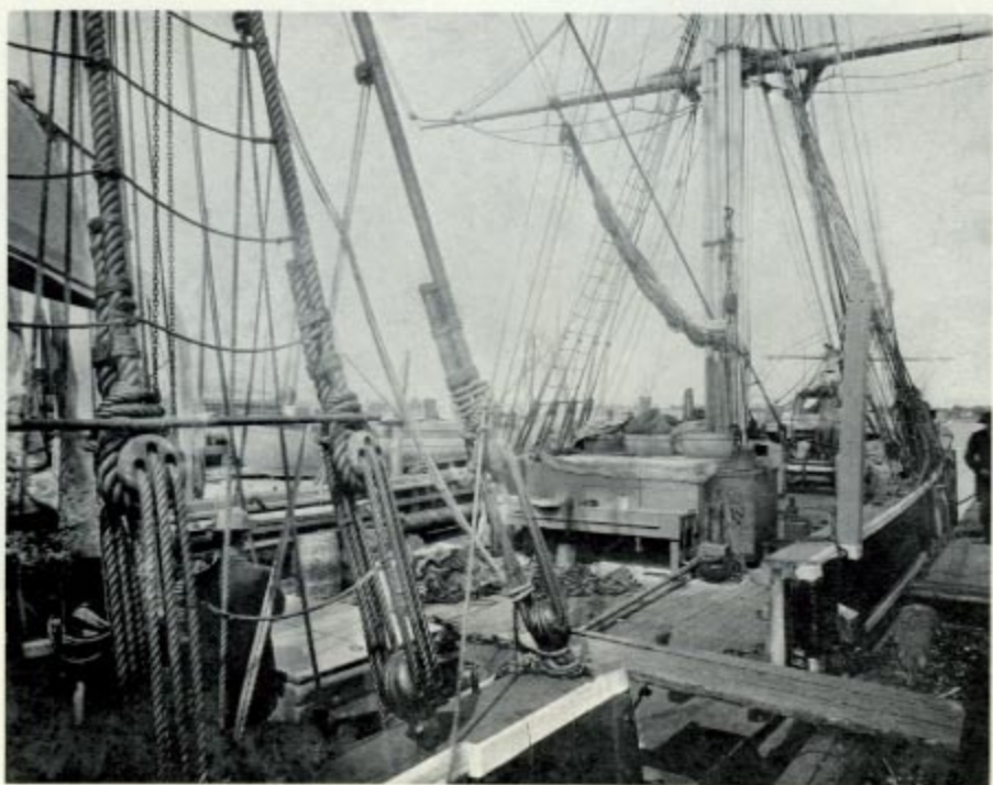
Bark Kathleen , 306 12/95 tons, built at Philadelphia, 1844. Shown at wharveside, fitting out
