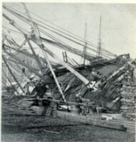
Unknown vessel hove down for recoppering, probably before 1860. The vessel's deck arrangement and fittings are characteristic of many early nineteenth-century whalers. Note the windlass abaft the foremast
