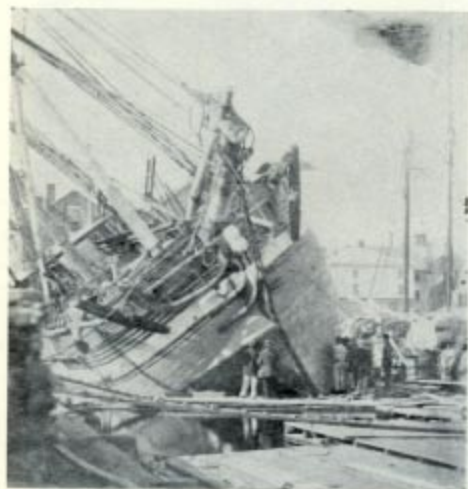
Unknown vessel hove down for recoppering, probably before 1860. The vessel's deck arrangement and fittings are characteristic of many early nineteenth-century whalers. Note the windlass abaft the foremast
